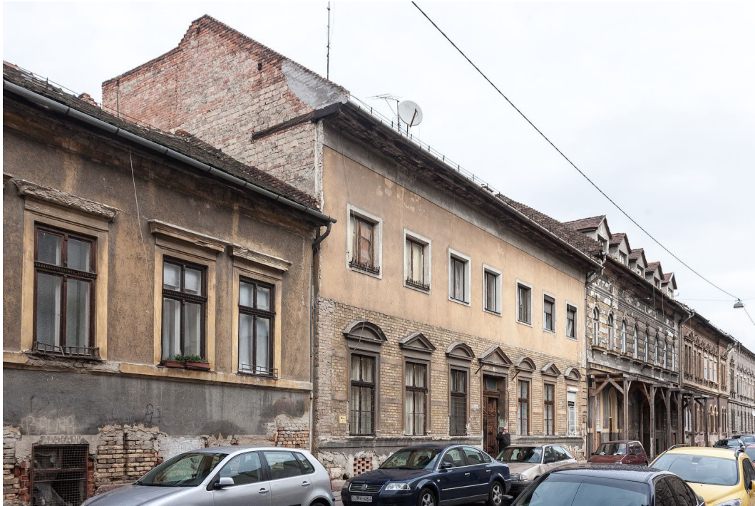
Photo 1. Typical 2-storey buildings in Orczy-district with ornate street façades. (source: 24. hu )
