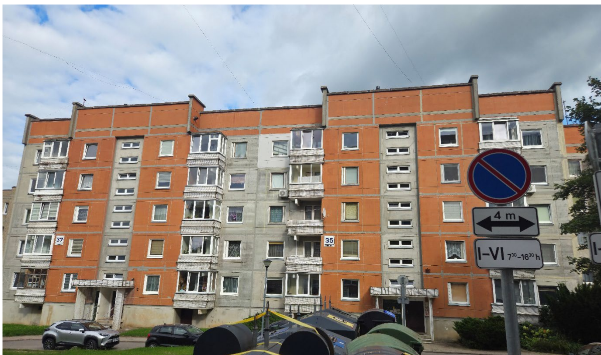
Figure 8. Examples of unrenovated buildings: a five-story multi-apartment building in Pergales 35, Elektrėnai.
