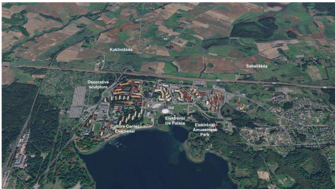
Figure 3: Overview of the pilot area and its surroundings, with selected buildings highlighted in beige, orange and red
