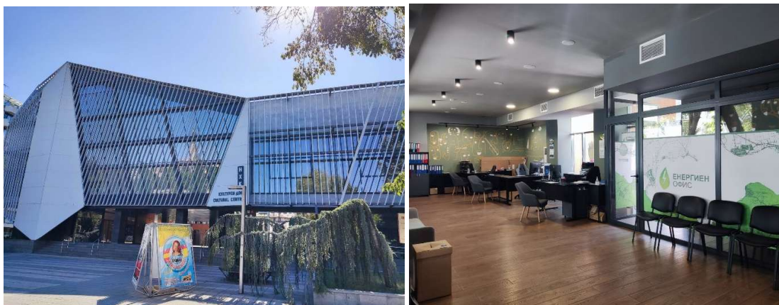
Picture 2. The building and the office of the RC in Burgas
